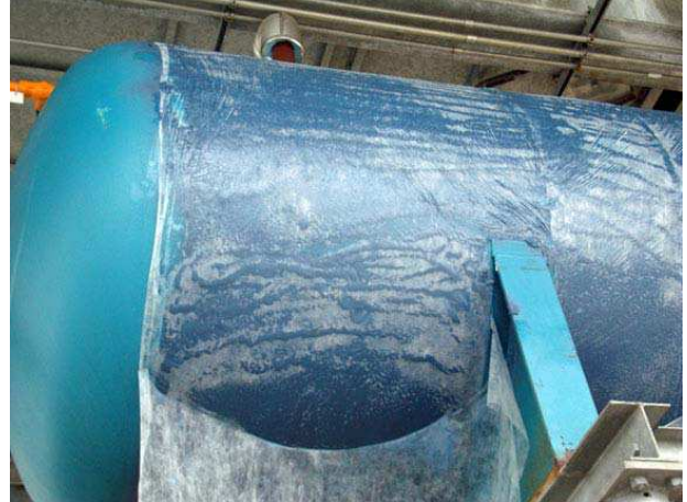
GeoWrap™ INSTALLED OVER RG
